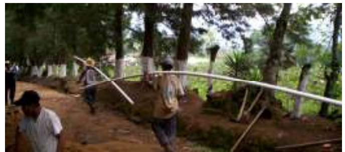
Yalu men taking new, donated pipes to install in the village
