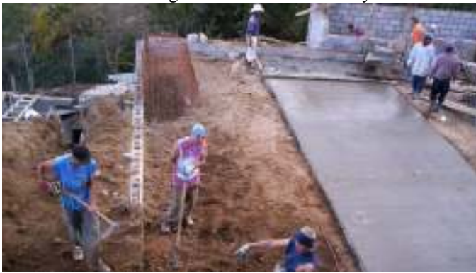
CAG students pouring concrete athletic court/patio
