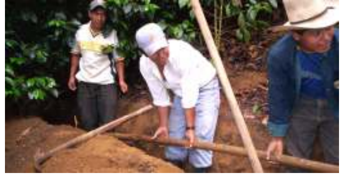
Removing 34-year-old pipe to improve clean water supply
