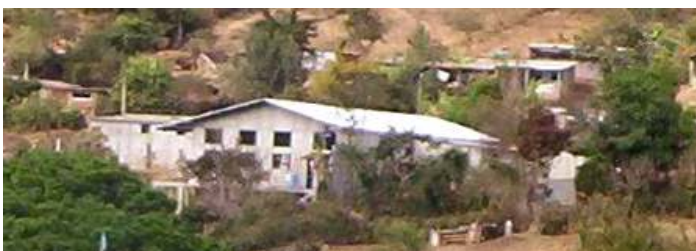
Feeding center view from across the Yalu valley February 2006
