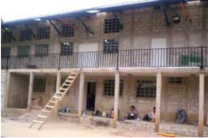
Yalu feeding center nearing completion
